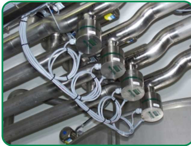
Fig. 2: Phase separation in the CIP return, using conductivity sensor ILM-2.
