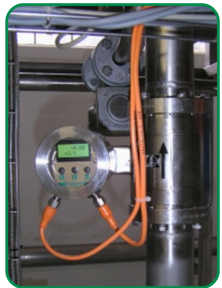
Fig. 1: The magnetic-inductive flowmeter, type FMA, in the feed of the CIP-system.
