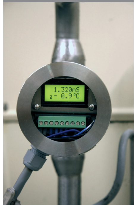
Fig. 2: Continuous conductivity measurement at the reaction tank with inductive conductivity meter ILM-2 from NEGELE
