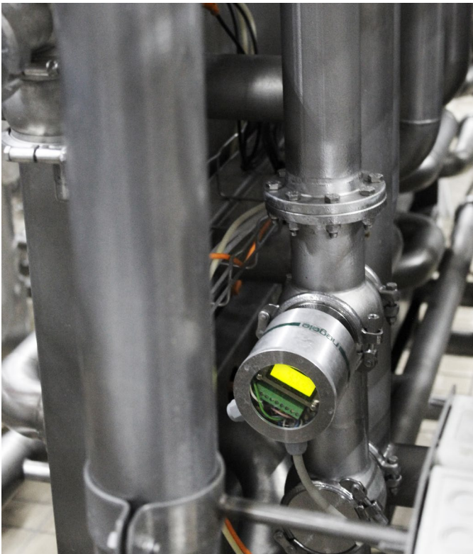
Continuous quality monitoring during keg filling (top) and canning (bottom) with the ILM-4. On the left image the ILM-4 for CIP acid/lye concentration control.
